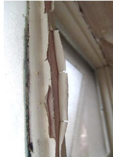
Fig 1. One of the major problems associated with timber use in outdoor applications – delamination of paint from the timber surface.
