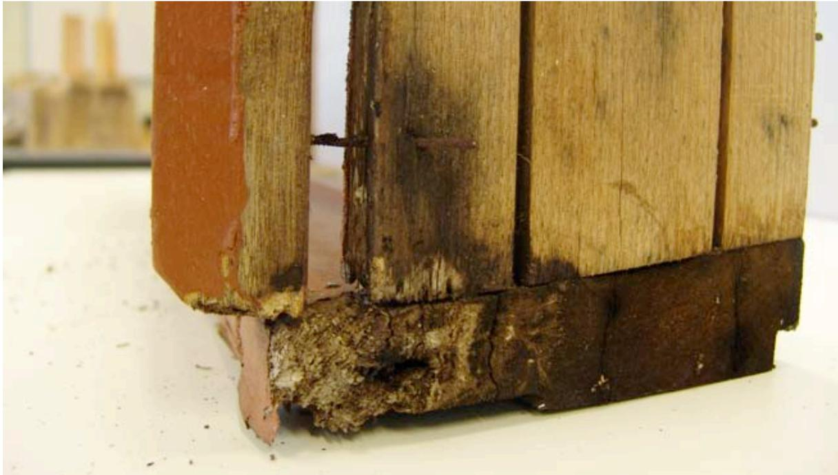
Fig 7. Timber deterioration between a weak butt joint due to water penetration.
