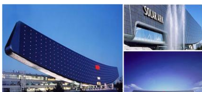
Figure 9. Sanyo Solar ark overall view
