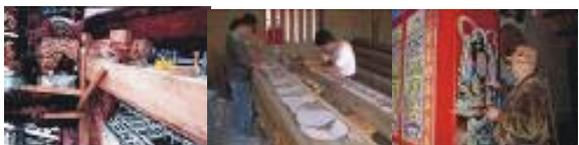
(Fig.4) Restoration of the decoration architecture: The left figure shows the wood carving restoration while the restoration for color painting is shown on the right.
